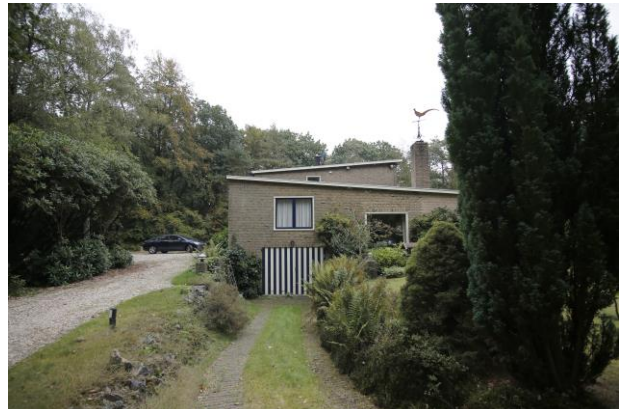
Entree in pandige garage
